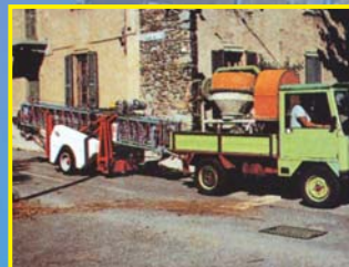
Traino in cantiere
